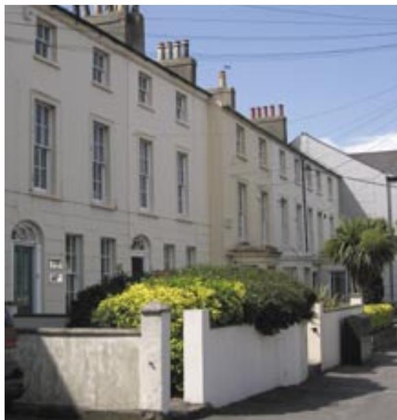
windows and eaves, chimneys several flues deep with corbelled detailing and double pitch dormers.
